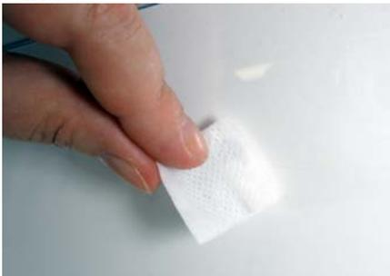
Figure 17. Adhesive Mount Antenna – Step 2. Peel Protection from Adhesive Strip
